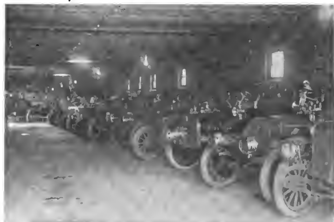
INTERIOR VIEW OF NEW LONDON GARAGE.
